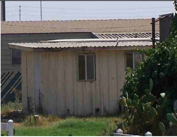
View looking southeast at shed (Building I).
