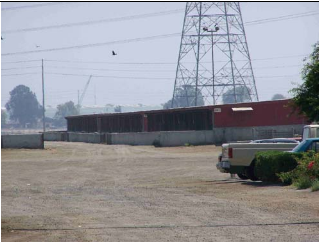
View looking southeast one of several hog pens (Buildings M).
