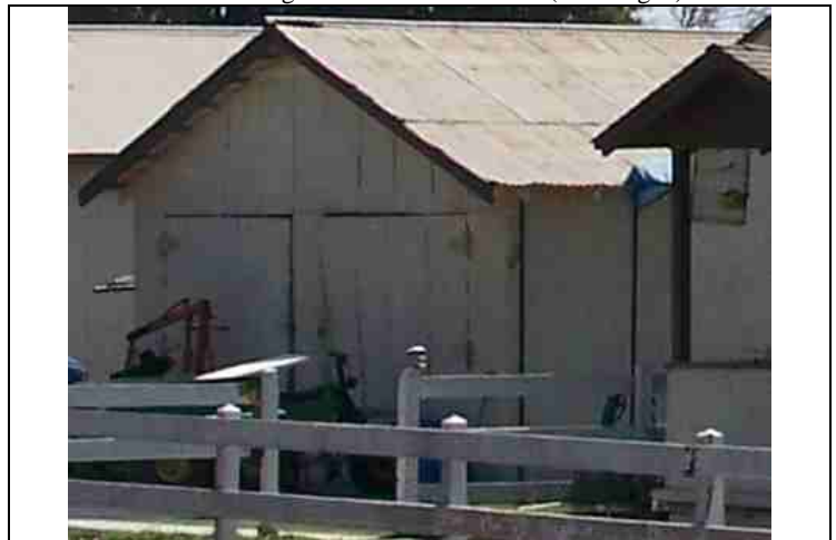
View looking southeast at 1947 garage (Building D).
