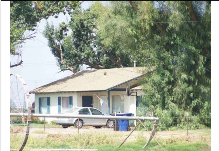
View looking northwest at Building D.
