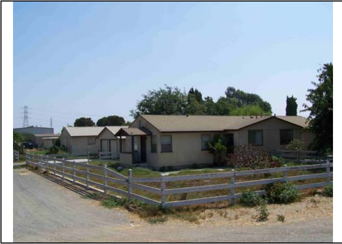
View looking southeast at 1947 SFR (Building A).
