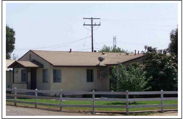
View looking southeast at 1947 SFR (Building B).
