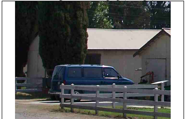
View looking southeast at 1947 building (Building F).
