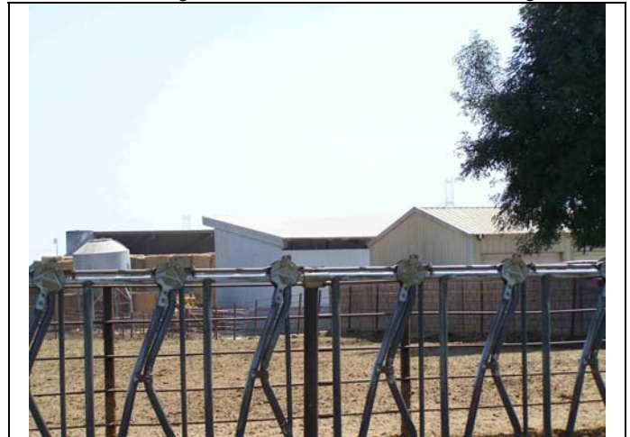
View looking southeast at Buildings C, which are seen at left.
