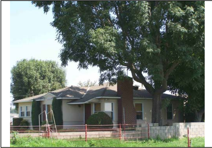
View looking northeast at south elevation of Building A.
