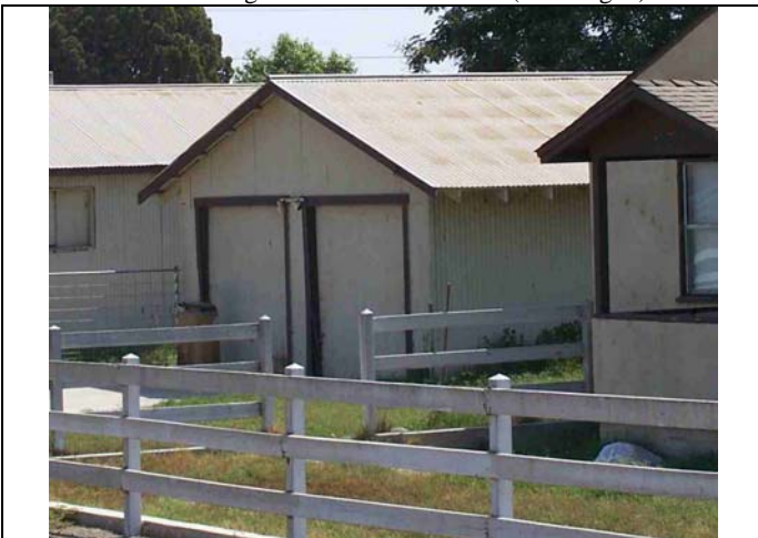
View looking southeast at 1947 garage (Building C).
