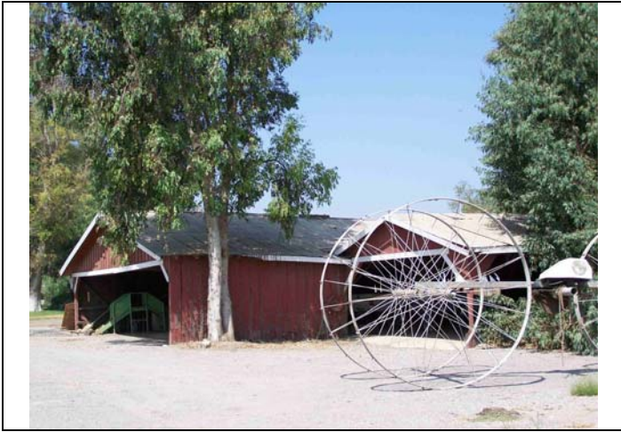
View looking northwest at Building B.
