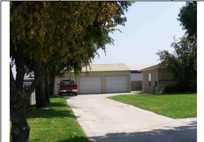
View looking southeast at Building B.
