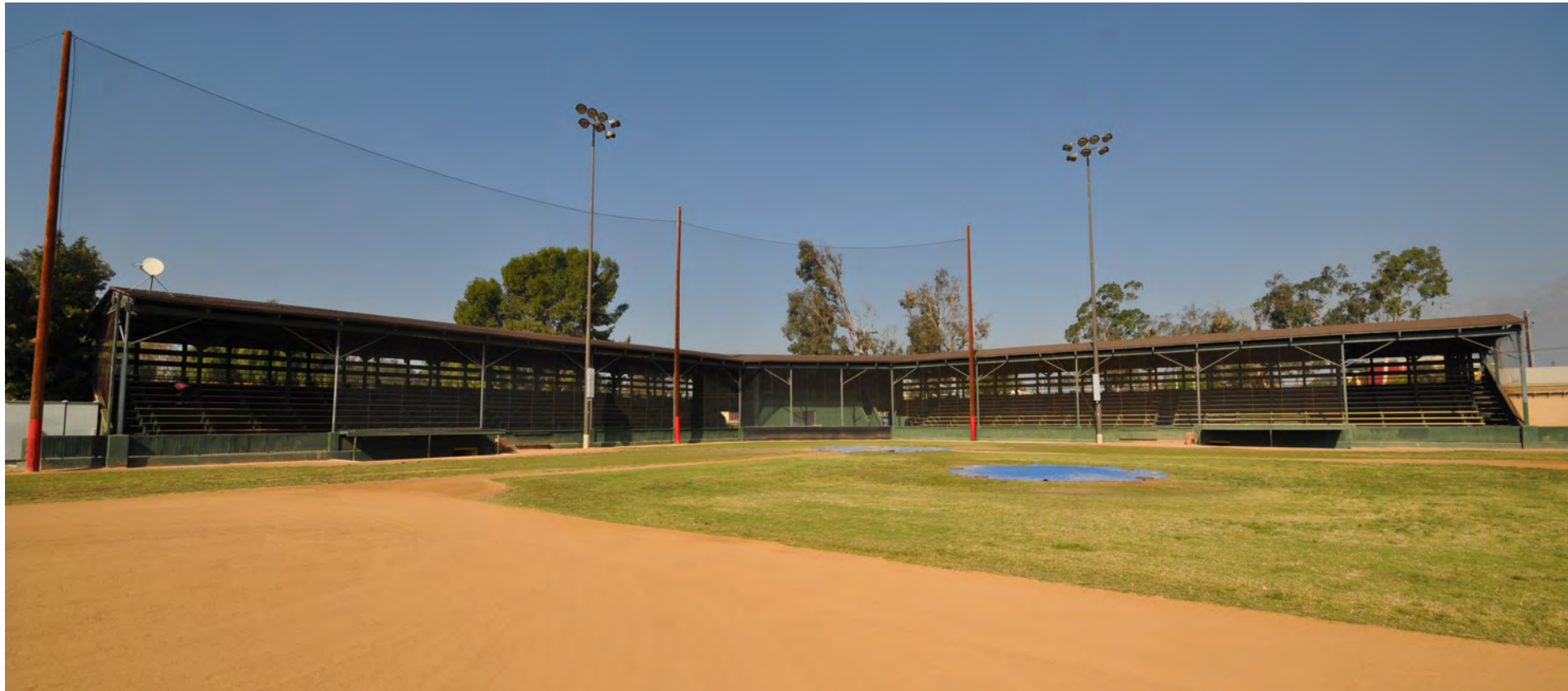
Figure 1. Jay Littleton Ball Park, looking northwest towards the grandstand.
