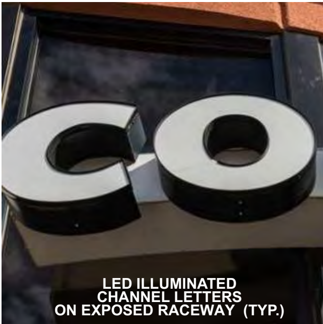
FACE & HALO LED ILLUMINATED BUILDING ADDRESS NUMERAL CHANNEL LETTERS (TYP.)
