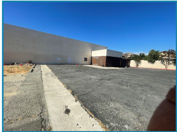
View Looking East (Side of Building)
