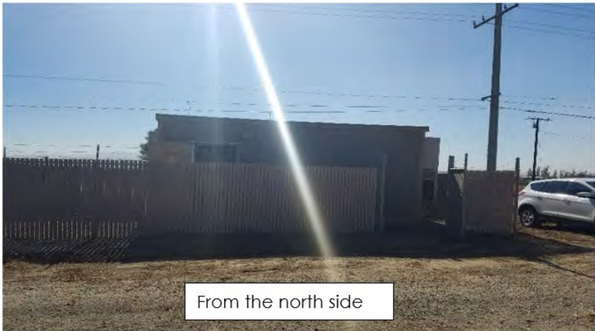
Existing Equipment Shelter and fencing
