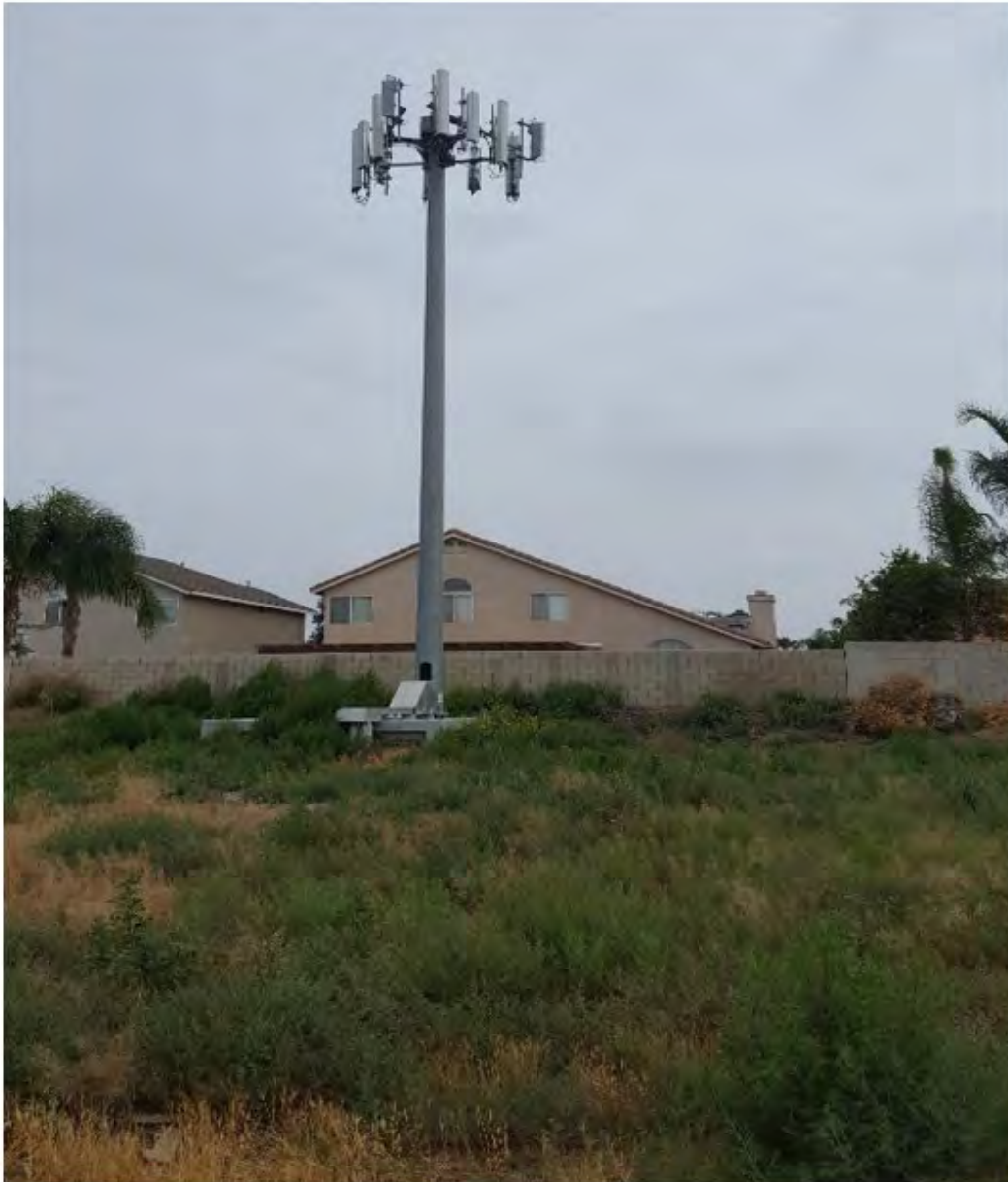
Temp Pole to be removed.
