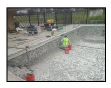
This project included plastering of the deteriorated pool surface which was chipping to extend the life of the pool surface by 10 to 15 years.
