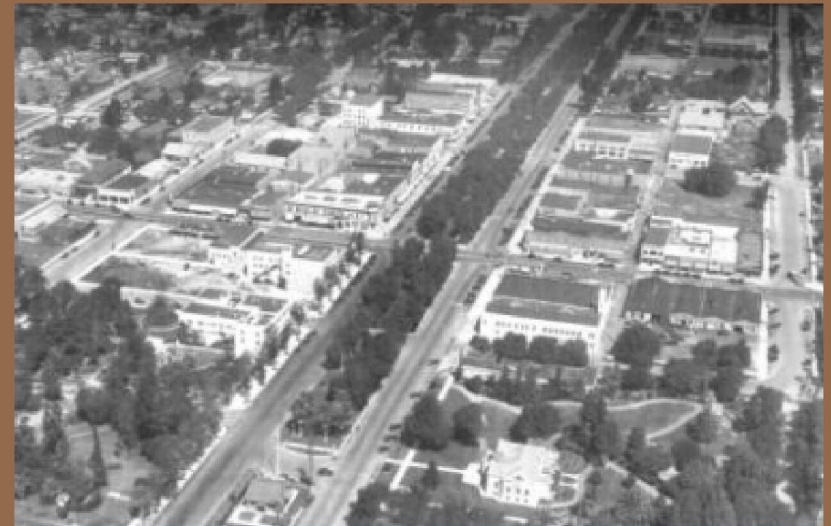
Euclid Avenue is a major scenario and historic resource in the city.
