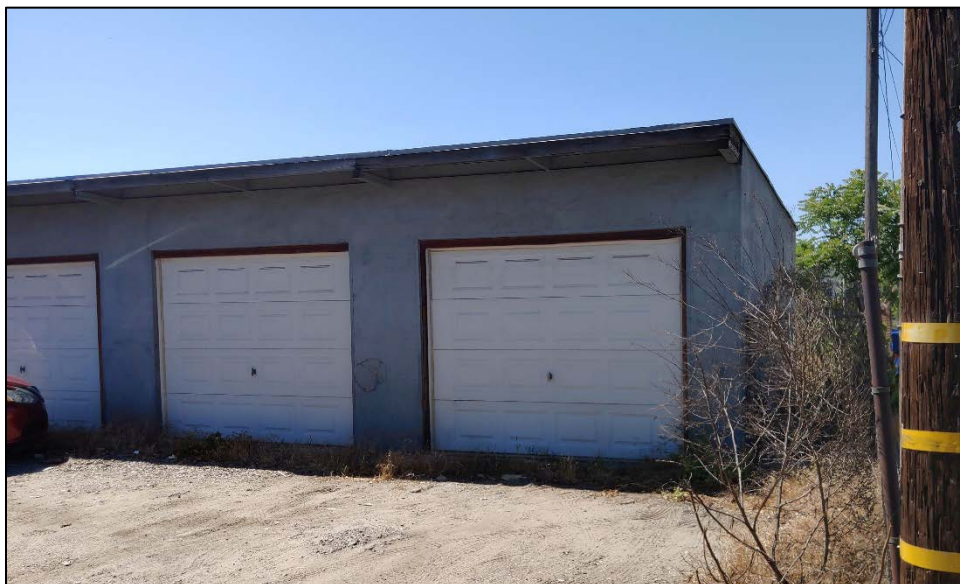
Detached 3-Car Garage – view looking southeast
