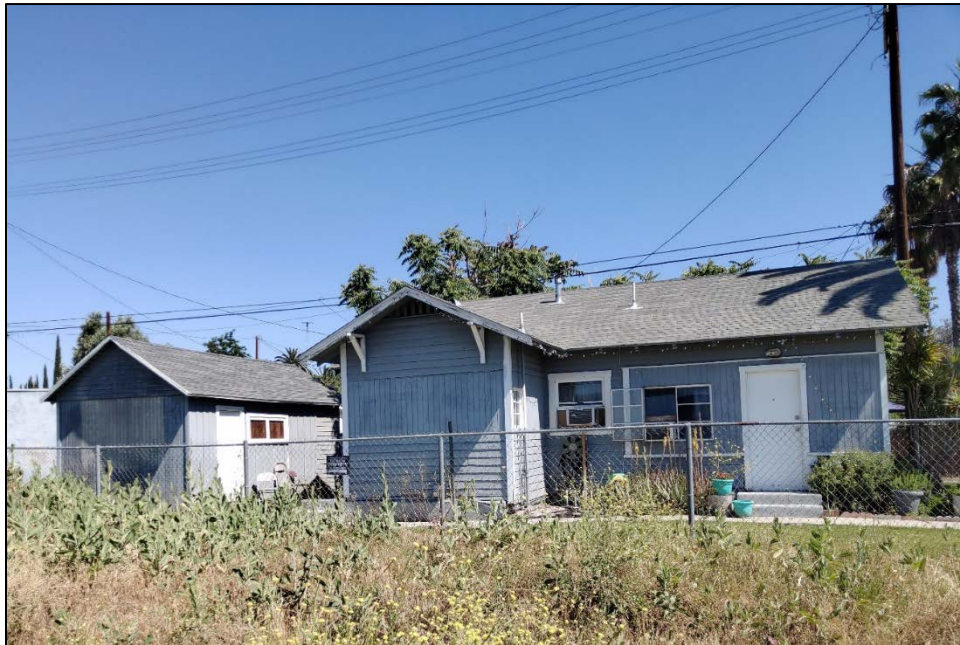
Residence and Detached One-Car Garage – view looking north
