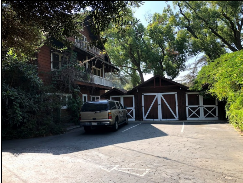
Figure 3: Graber House. Northeast Elevation and Garage
