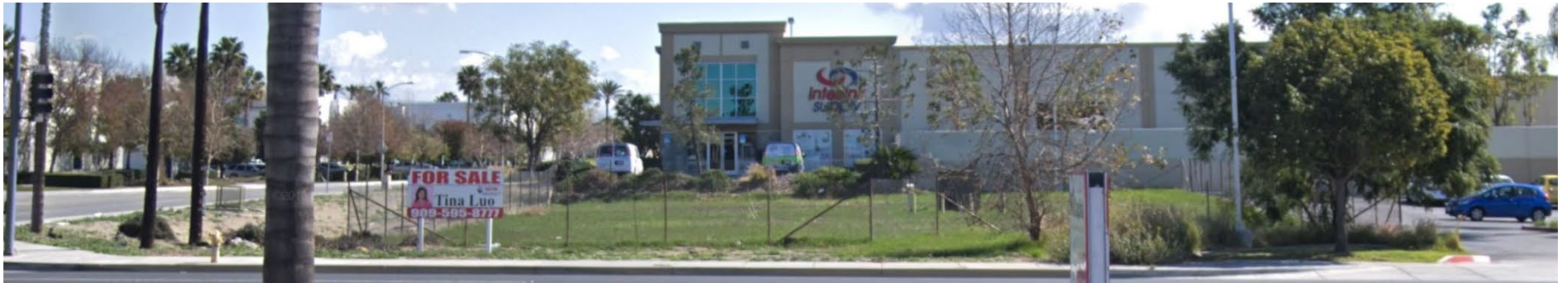
VIEW LOOKING EAST FROM GROVE AVENUE
