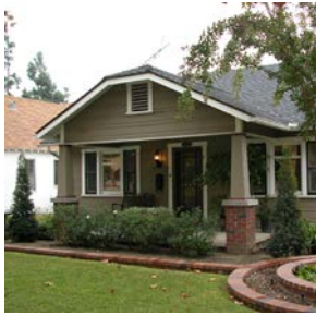
Covered porch with distinctive gable end treatment.
