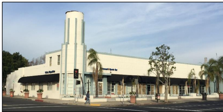
Figure 2 (Above): Site – View looking northwest
