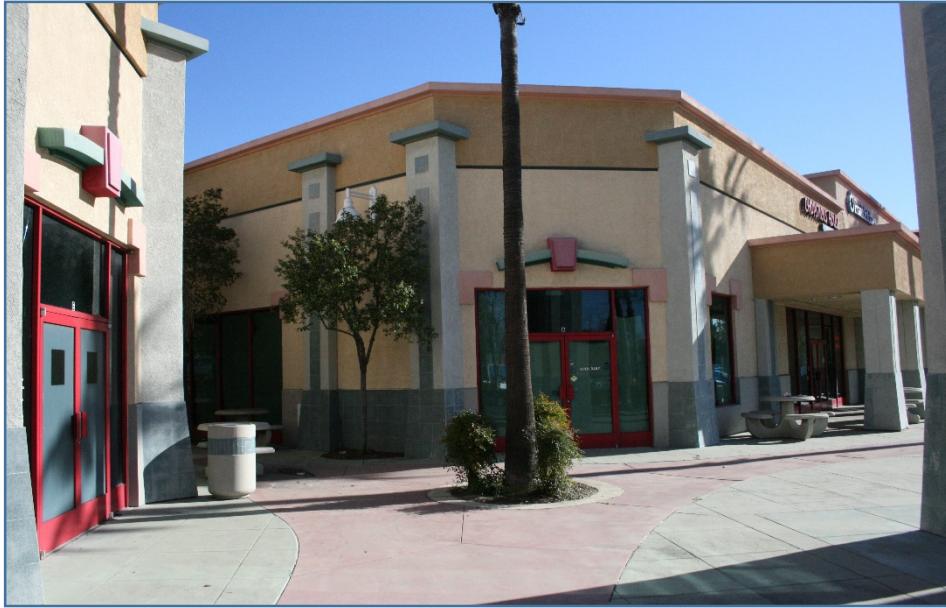
Above: View of South Elevation (Entrance)
