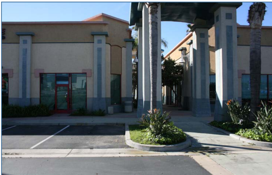
Above: View of North Elevation (Rear Entrance)
