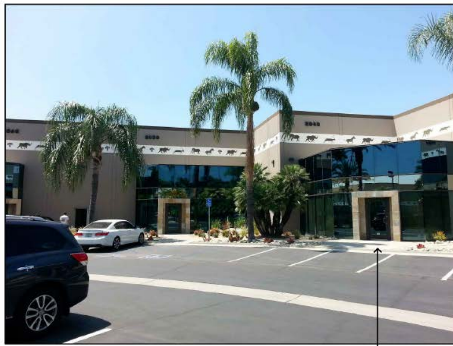
Southwest View of Building's Main Entrance
