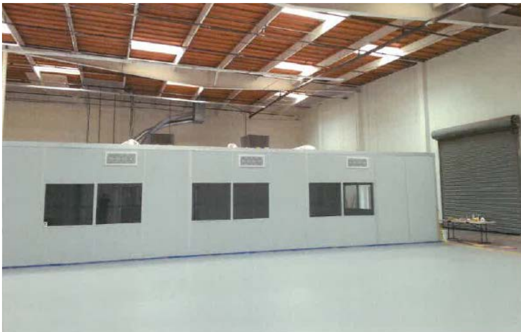
OUTSIDE VIEW OF 2,220 SF CLEAN ROOM
