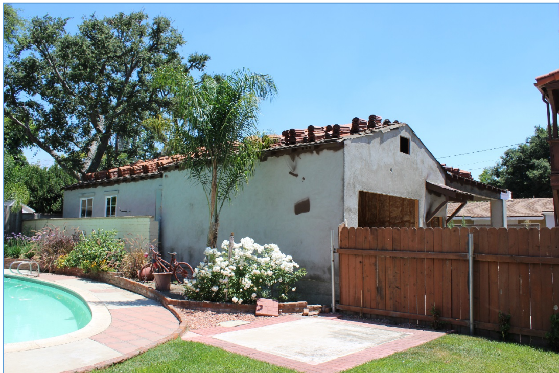
Below: West View
