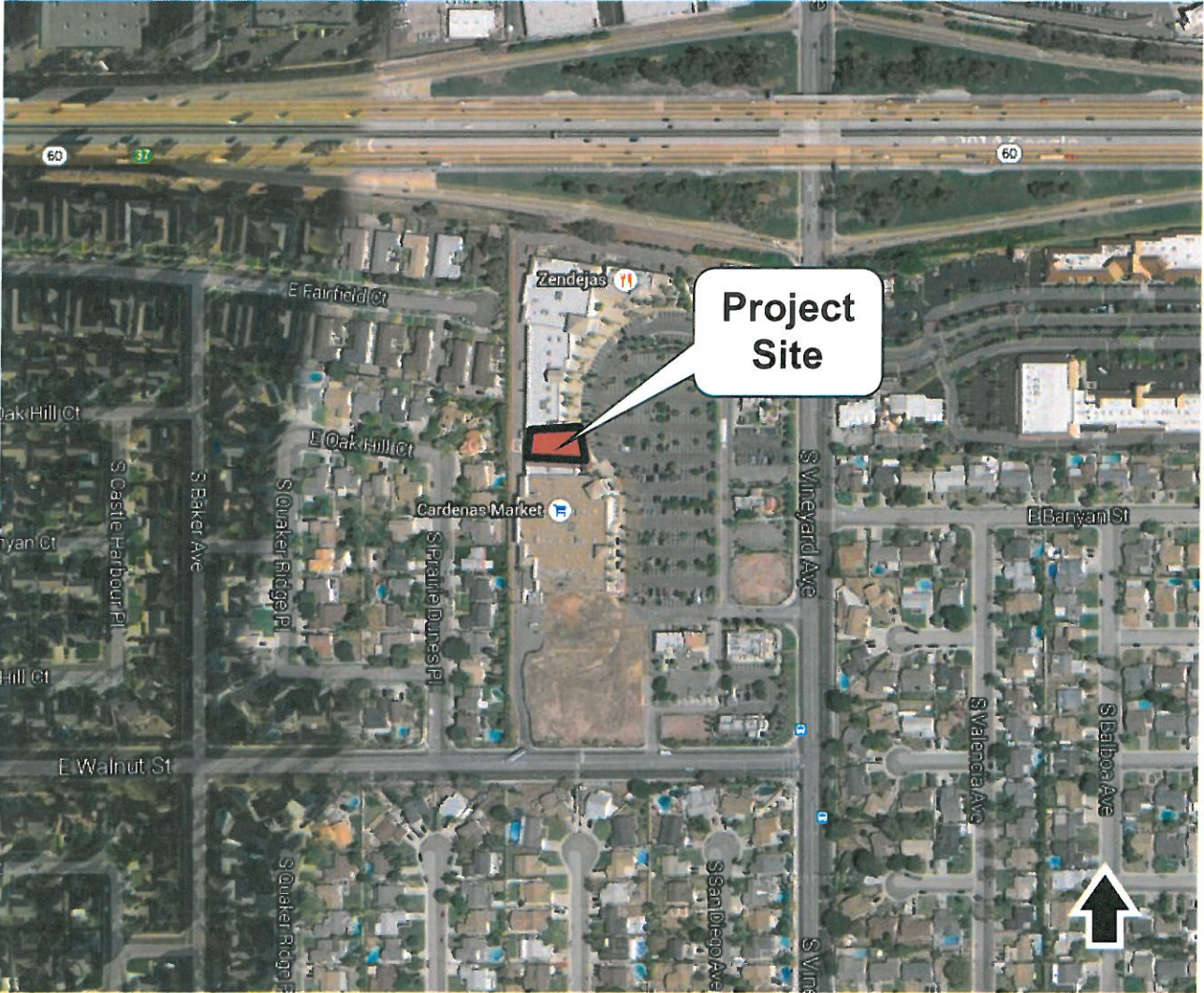
Exhibit A: Project Site Aerial
