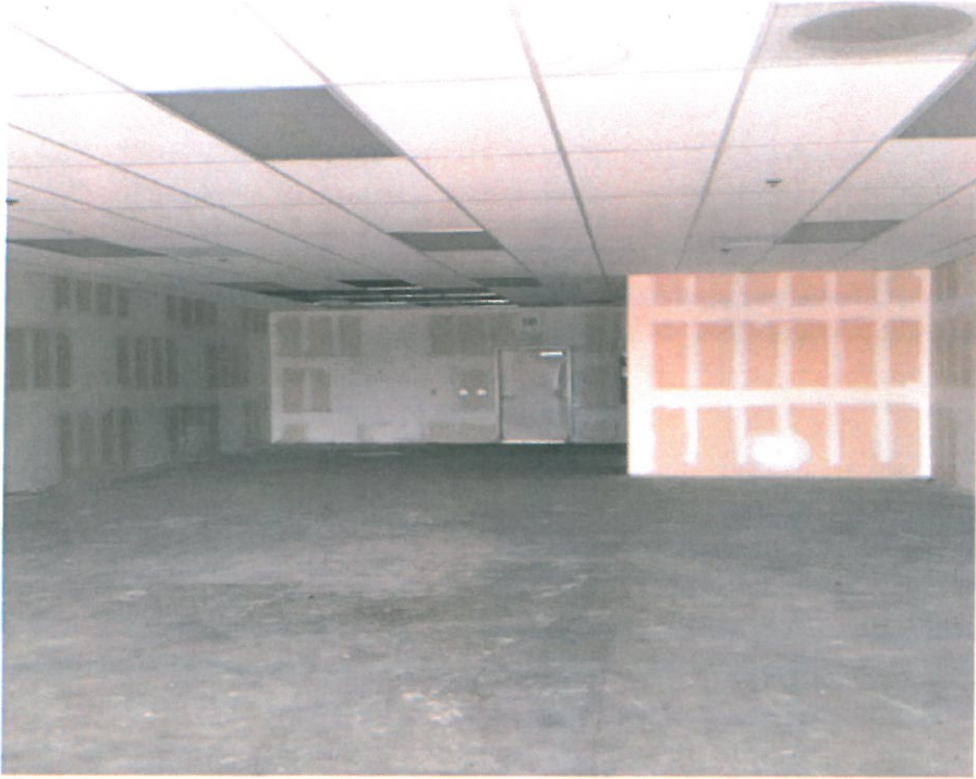
Project location, interior.
