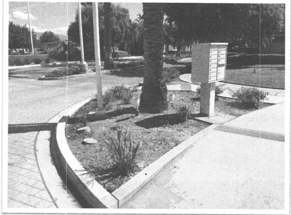
Area Missing Landscaping
