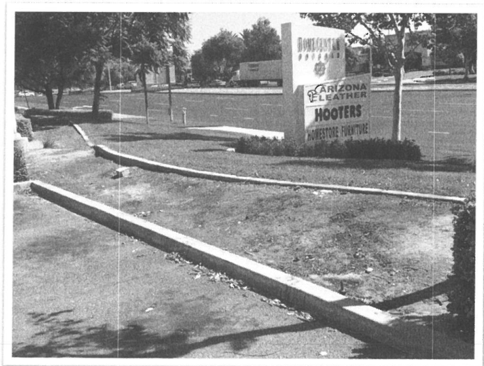
Missing Landscaping Areas
