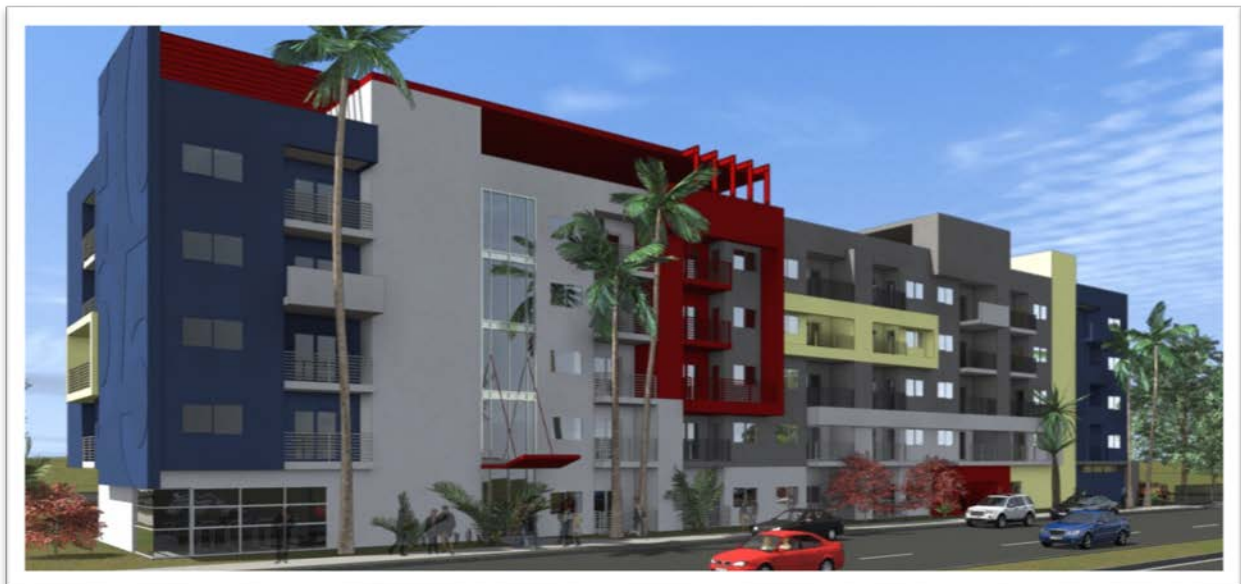
Close-Up of North Elevation
