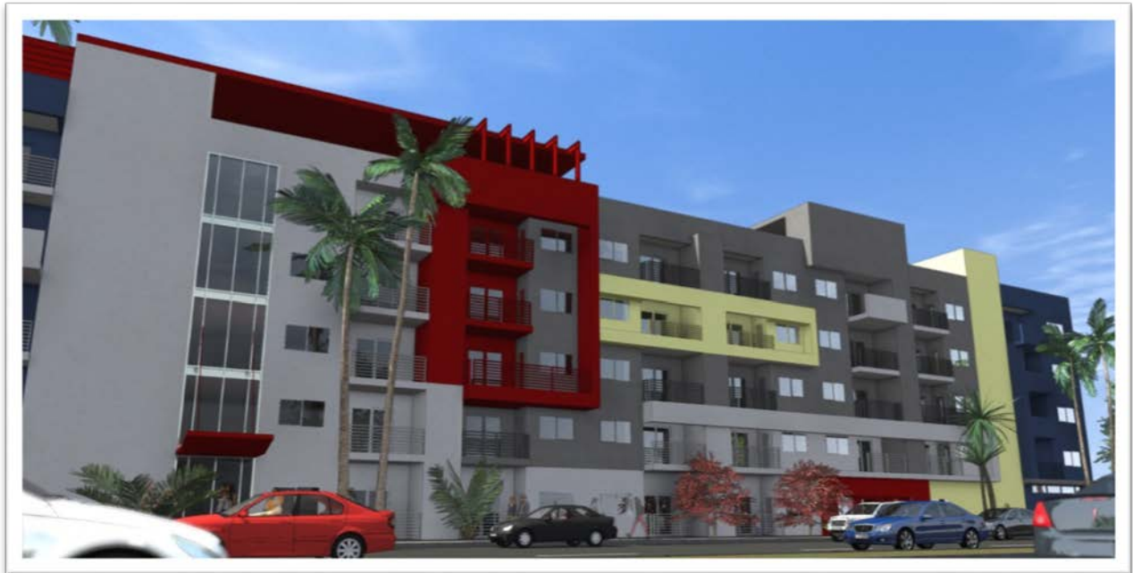
Close-Up of North Elevation
