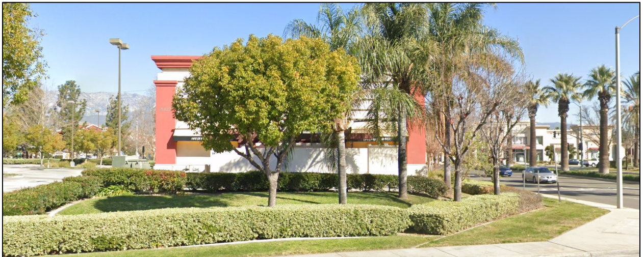
South Elevation (Facing North)
