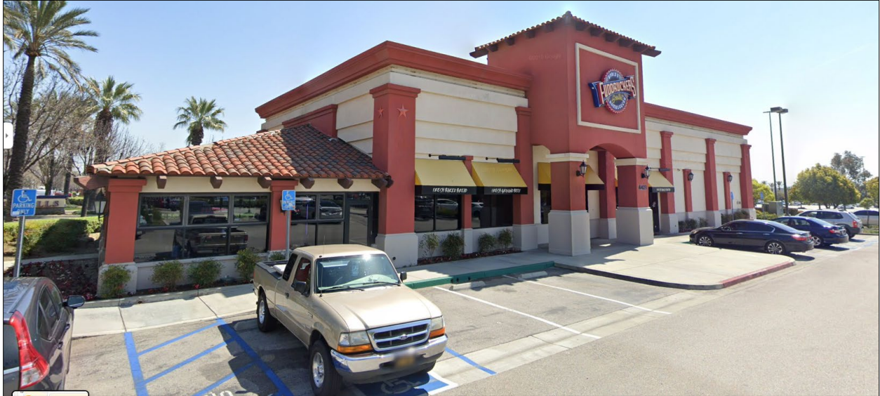
West Elevation (Front – Facing Southeast)
