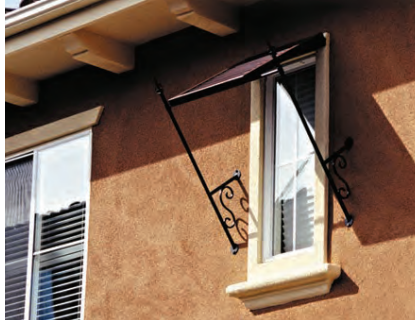
VERTICAL WINDOWS WITH WROUGHT IRON DETAIL
