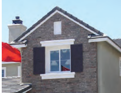
BRICK SIDING AND VERTICAL MULTI-PANED WINDOWS
