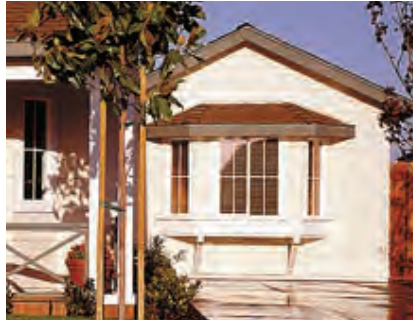
MULTI-PANE BAY WINDOW HORIZONTAL LAPPED SIDING
