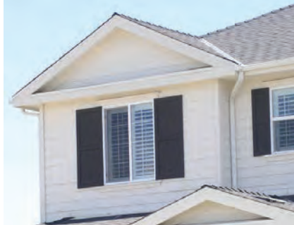
CLOSED PEDIMENT AND SHUTTERED WINDOWS
