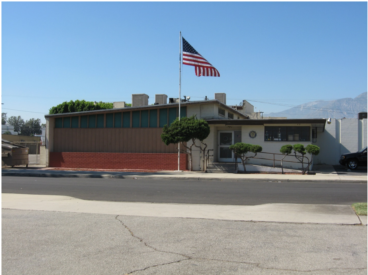
American Legion Building- 310 West Emporia Street- Tier III
