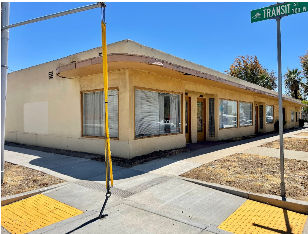
Office Building- 201-215 S. Fern Ave- Tier III
