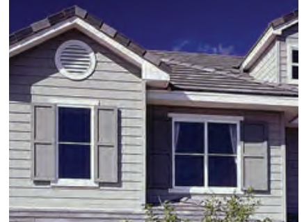
VENTED GABLE AND HORIZONTAL SIDING
