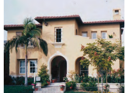
STUCCO WALLS WITH ARCHED OPENINGS
