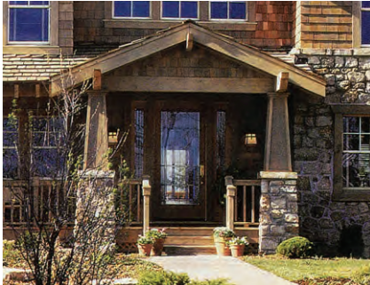
FRONT PORCH WITH BATTERED COLUMNS
