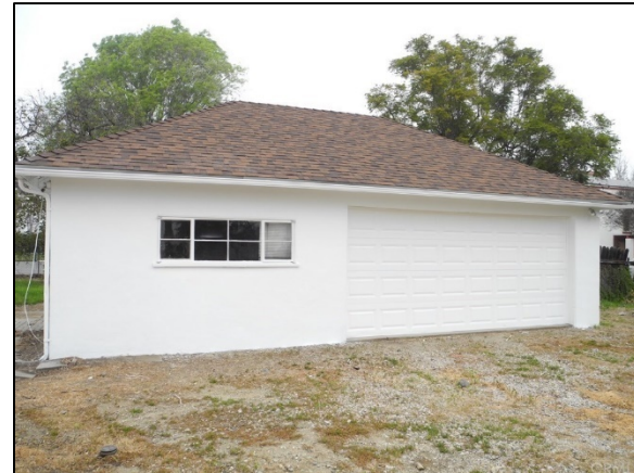
Detached garage with workshop View looking north
