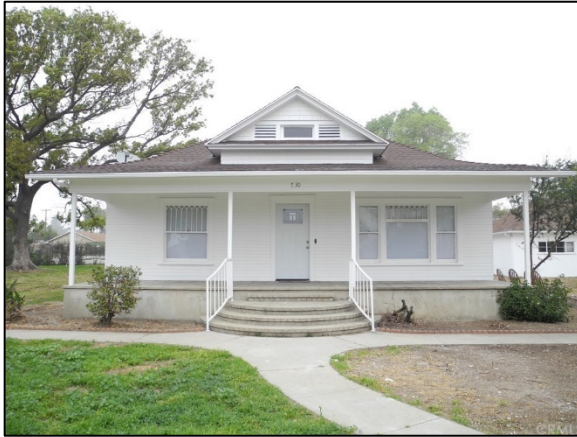
Residence-Front View looking north
