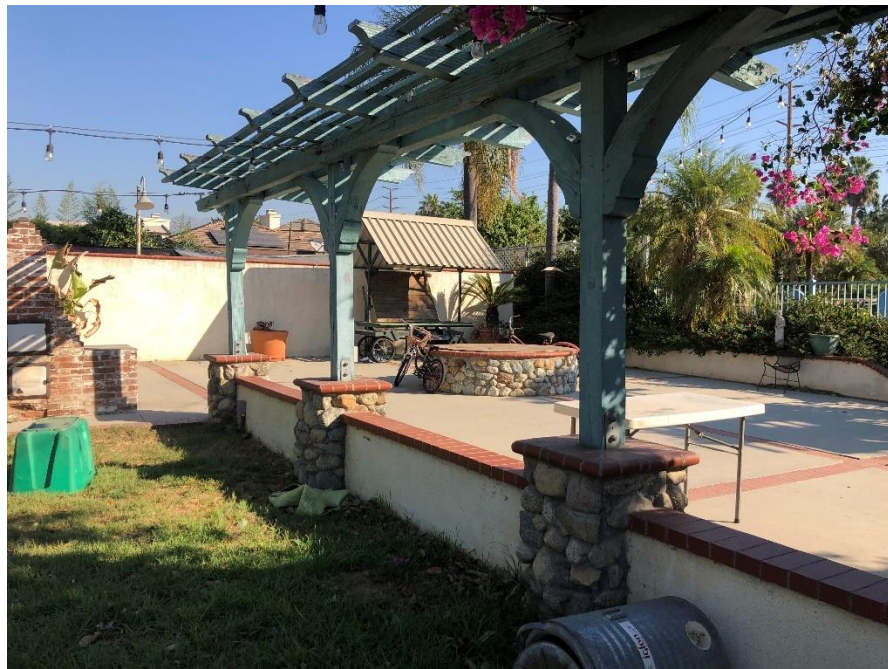
Figure 14. Concrete Patio (view northeast), 2112 S. Oaks Avenue SOURCE: Sapphos Environmental, Inc., 2020
