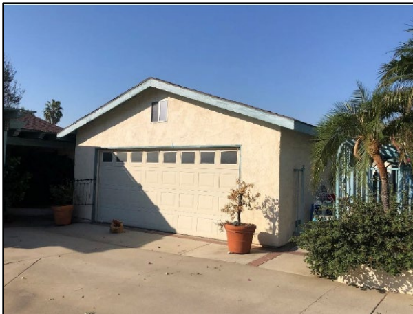
(No.2 ) Detached Garage –West Façade
