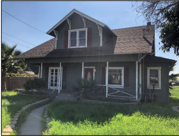
Single-Family Residence North Elevation
