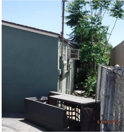
Western Façade, Garage, 1445 W. Mission Boulevard SOURCE: Sapphos Environmental, Inc., 2018
