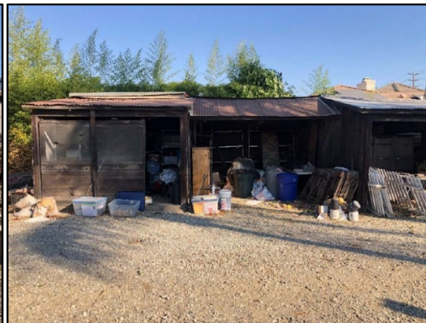
(No.5) Auxiliary Building 1
