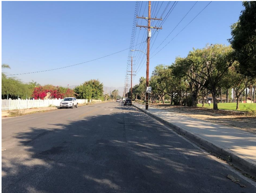
Figure 1A. Setting (view north), S. Oaks Avenue SOURCE: Sapphos Environmental, Inc., 2020
