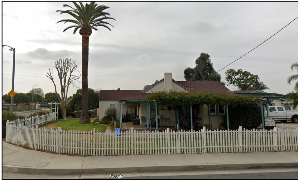
(No.1) Main Residence East elevation – view looking west
