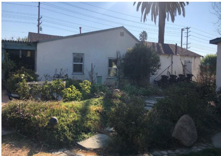
Figure 8. Western Façade (view southeast), 2112 S. Oaks Avenue SOURCE: Sapphos Environmental, Inc., 2020
