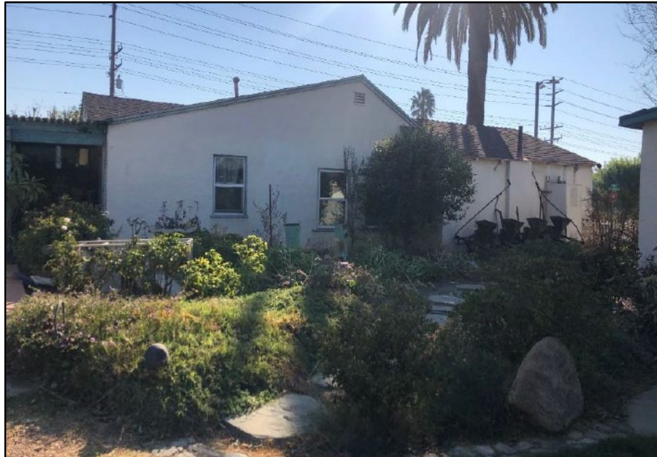
(No.1) Main Residence West elevation – view looking west
