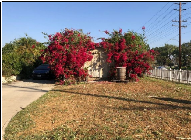
(No.3) Detached Garage –South Façade
