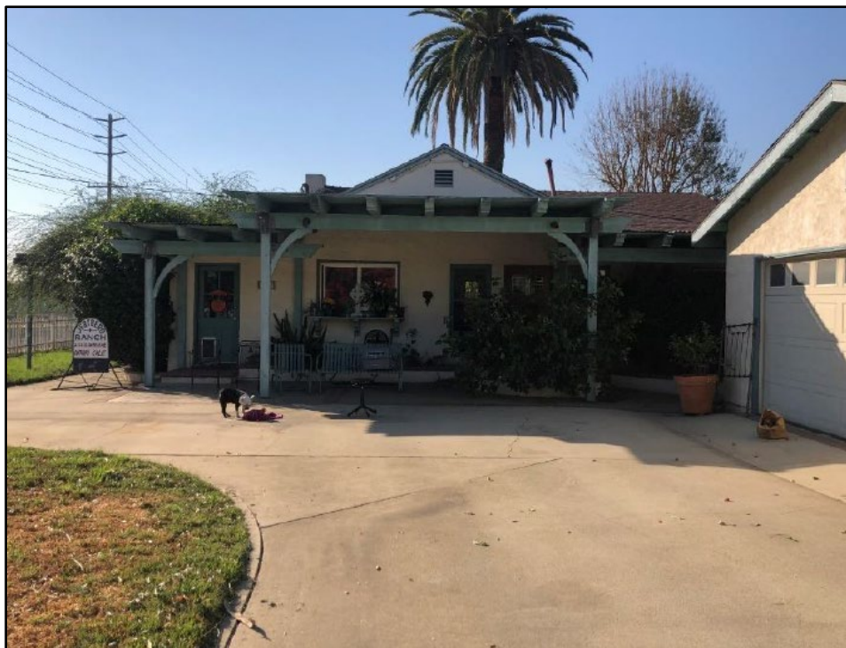
(No.1) Main Residence North elevation – view looking south
