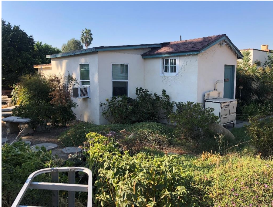
Figure 12A. Ancillary Building No. 2 (view southwest), 2112 S. Oaks Avenue SOURCE: Sapphos Environmental, Inc., 2020
