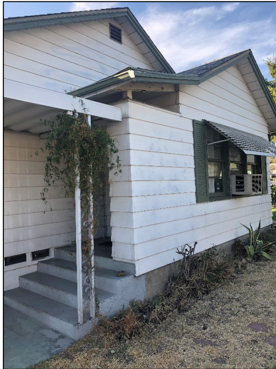
East elevation – view looking northwest
