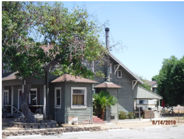
Western Façade, 1445 W. Mission Boulevard SOURCE: Sapphos Environmental, Inc., 2018
