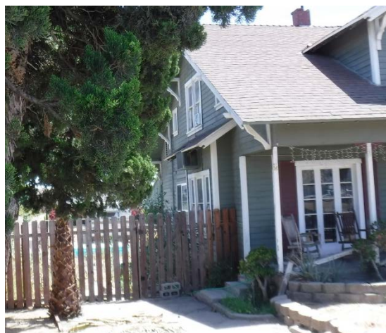
Western Façade, 1445 W. Mission Boulevard SOURCE: Sapphos Environmental, Inc., 2018
