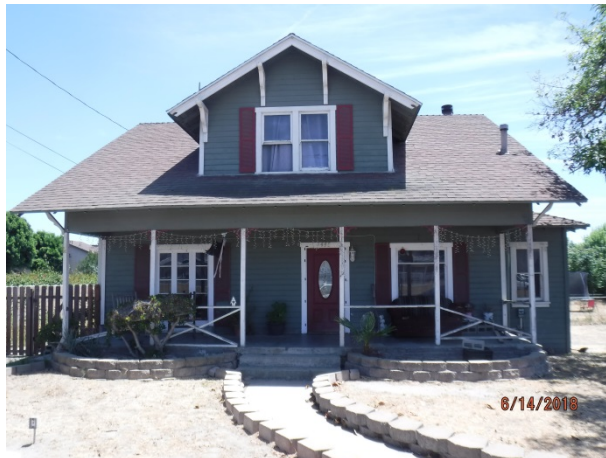
Primary Façade, 1445 W. Mission Boulevard SOURCE: Sapphos Environmental, Inc., 2018
