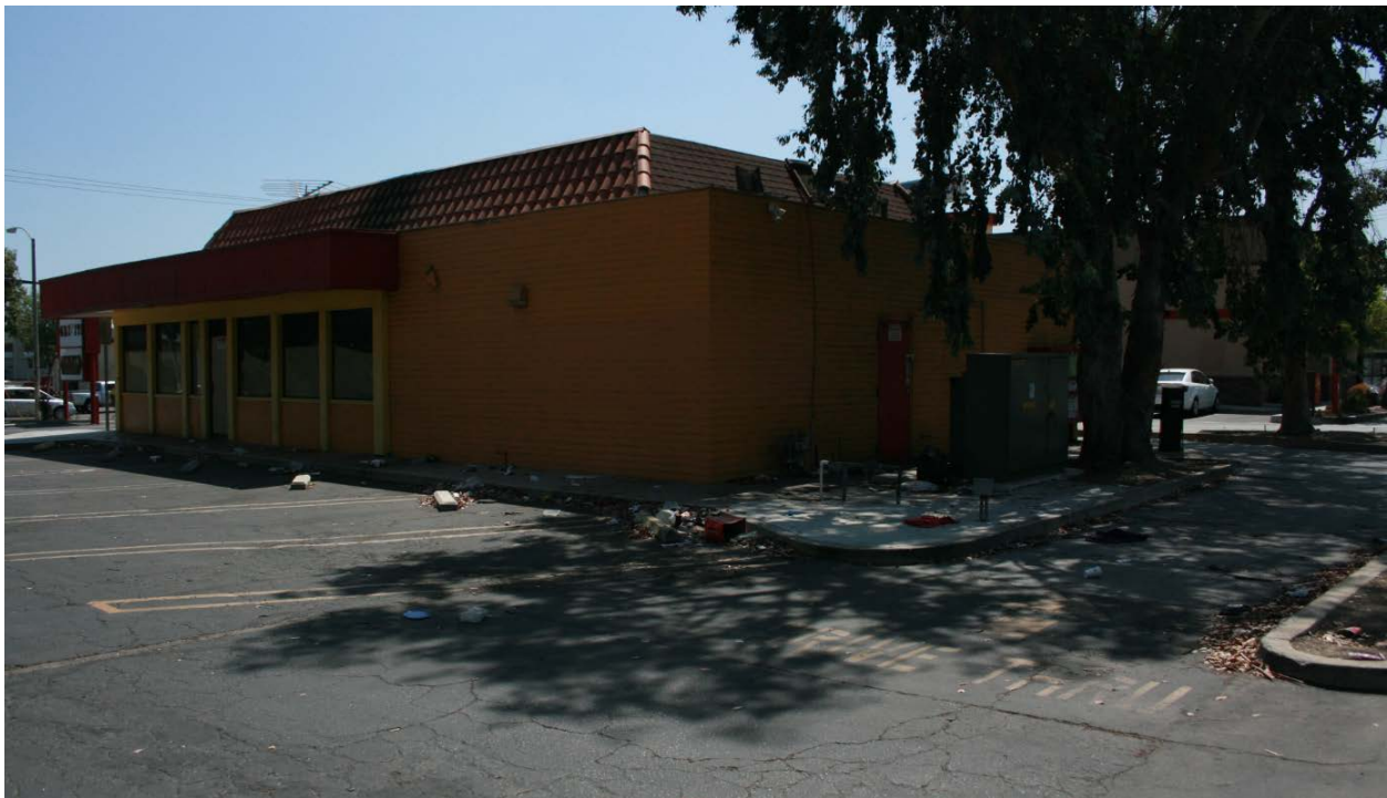
View of the northeast corner of building and existing drive-thru location
