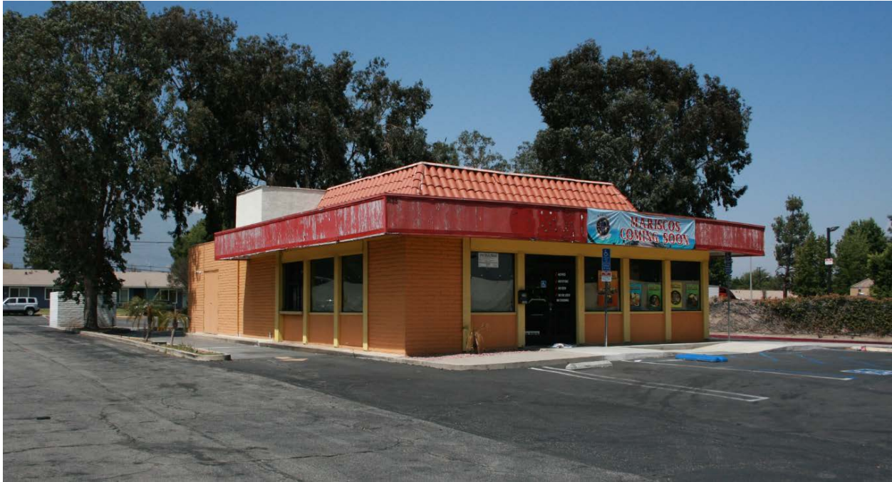
View of the Southwest corner of existing building and main entrance
