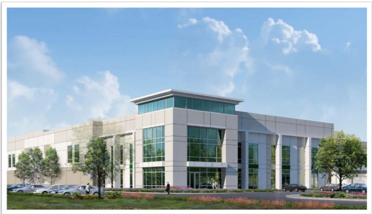
Figure 6: Typical Office Storefront
