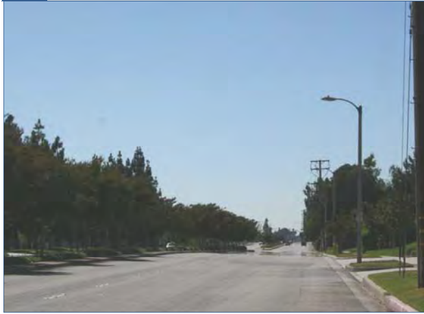
CCC Looking West on 6th St at Cleveland Ave Intersection
