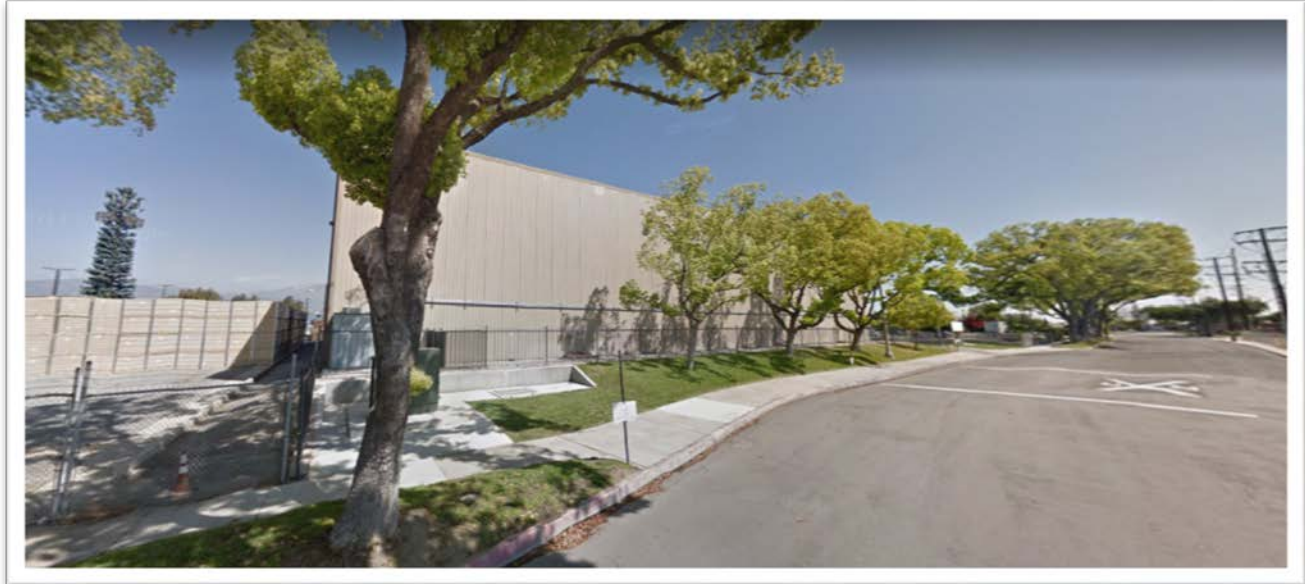
View of Project Site Looking East from Sunkist Street
