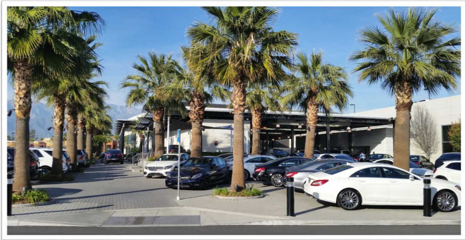
South Views of Existing Service Writer's Office and Shade Canopy
