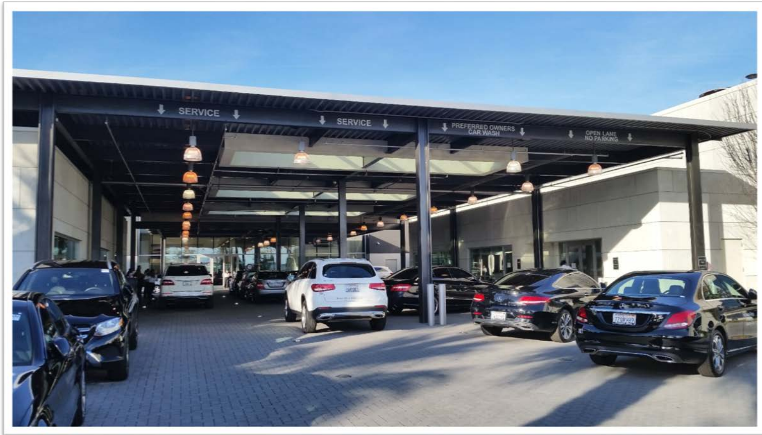
View of Front (South Elevation) of Existing Service Drive Canopy
