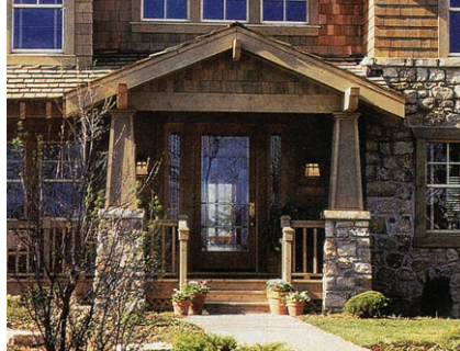
Front Porch with Battered Columns
