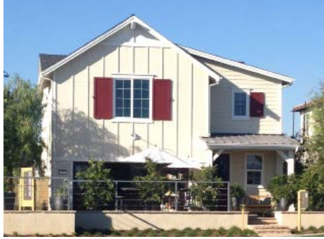
Board and Batten Siding
