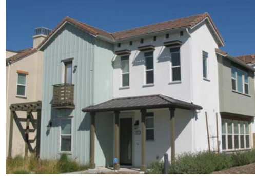
Proper Terminate Points for Siding and Color Accents
